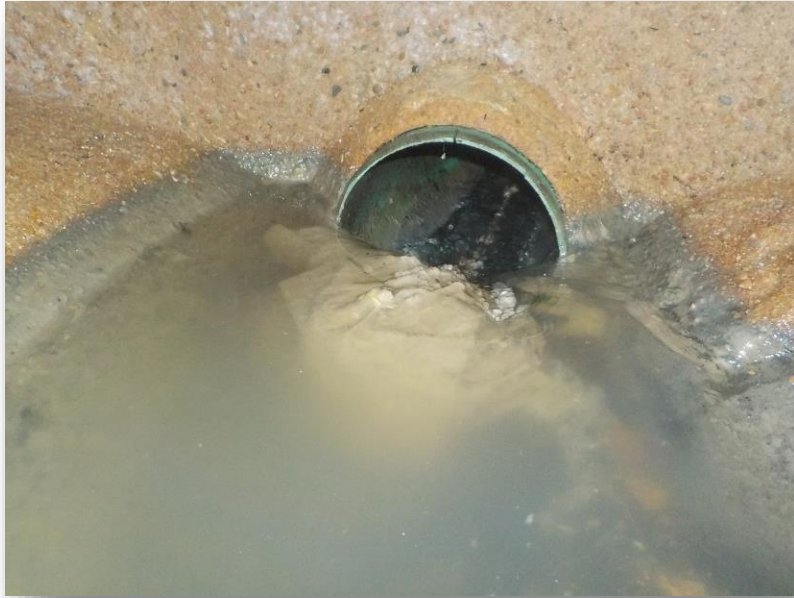
Stick Blocking Outlet Pipe Resulting in Ragging
