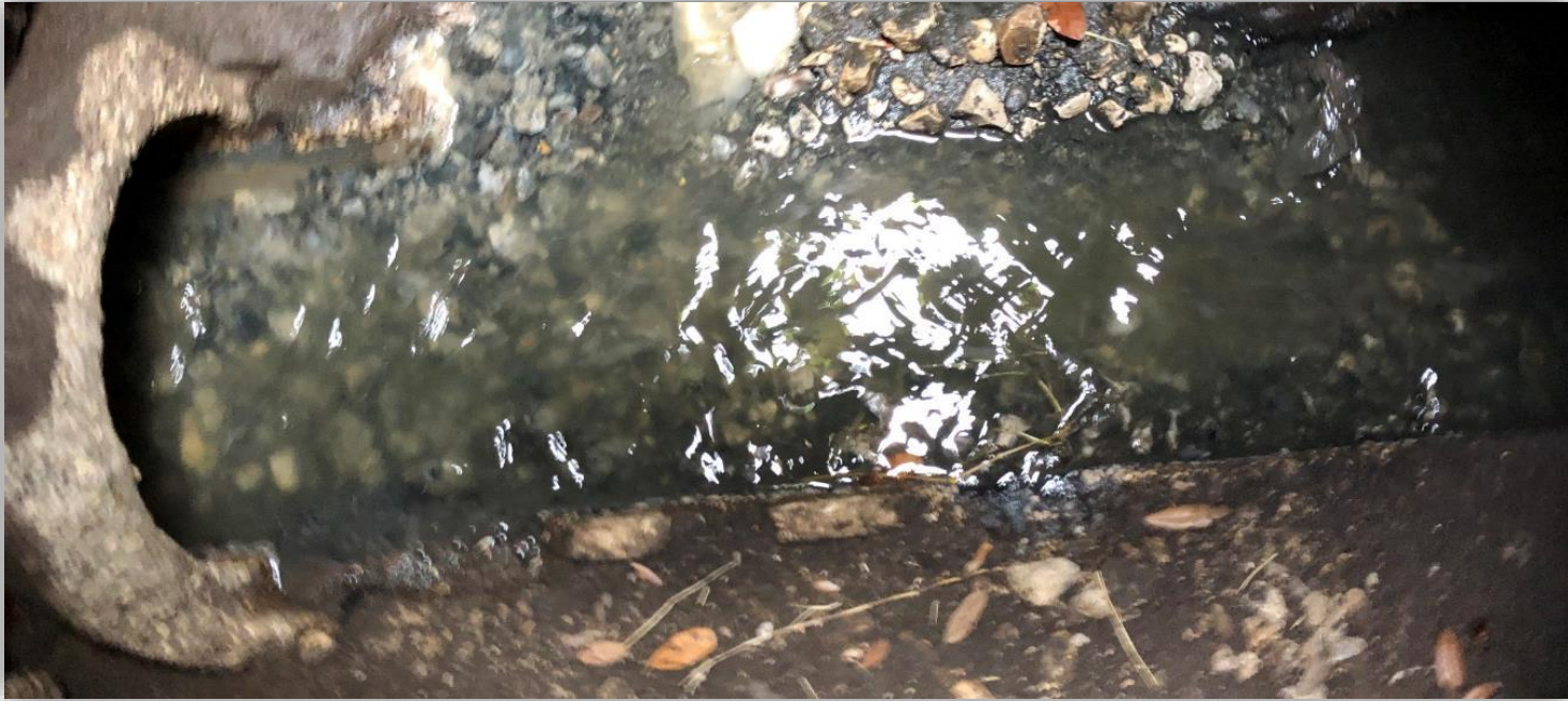
Gravel and Rocks Observed in Manhole Channel
