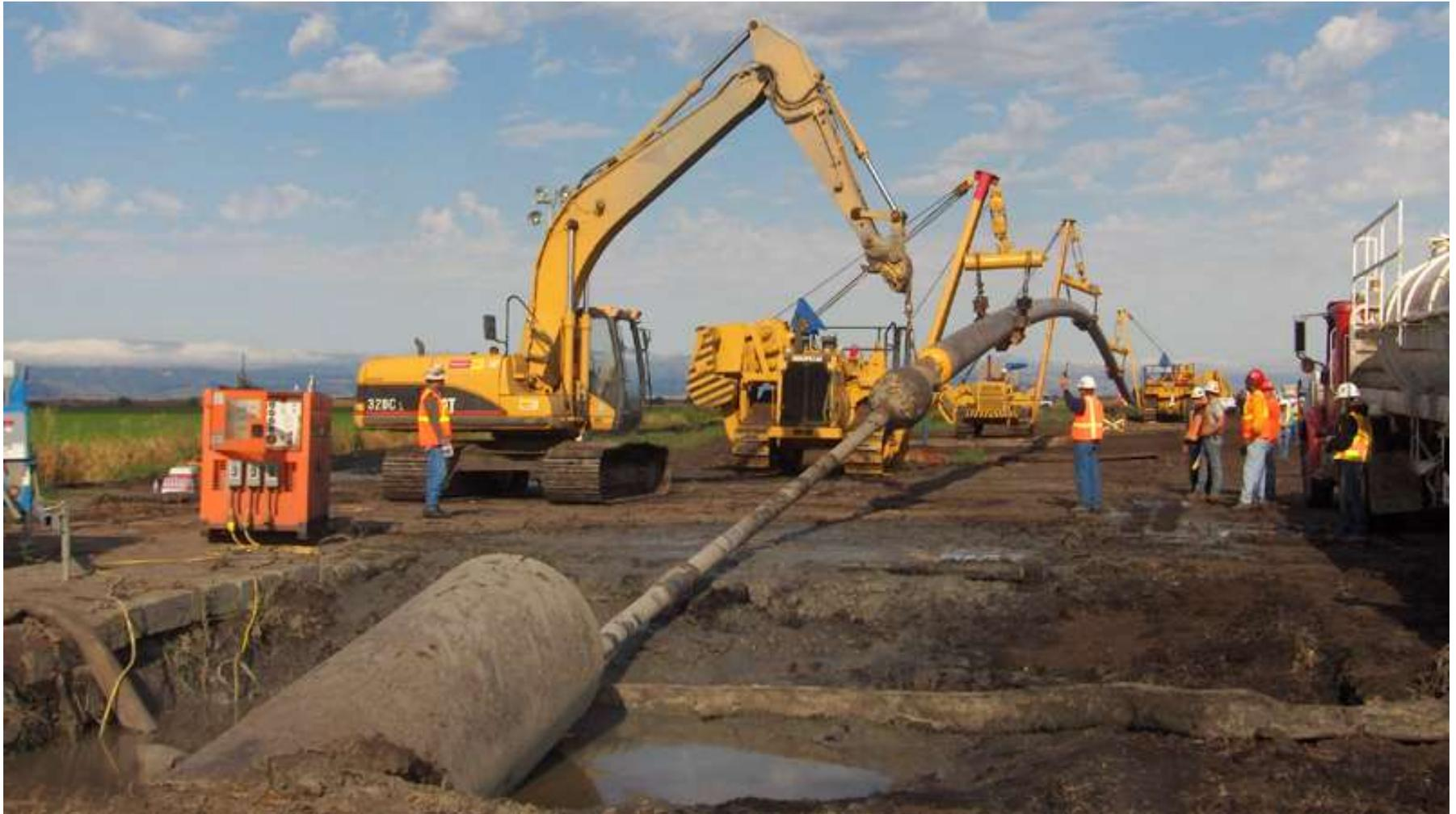
HDD Pullback Site – Large Diameter ( $\geq 24''$  OD)
