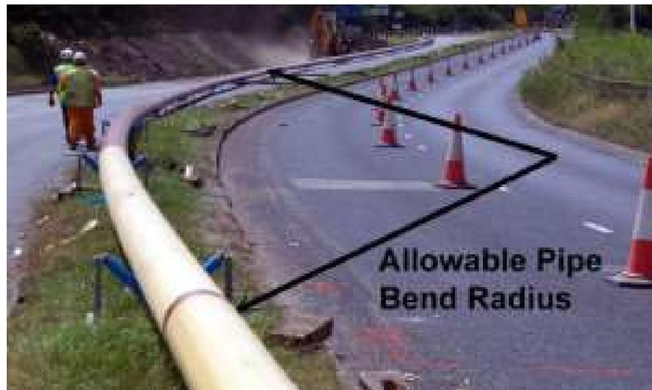
$R_{allow}$  → Material Bending Stress + Axial Stress due to Tension + Critical Ring Buckling
