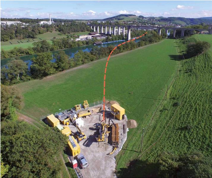
Horizontal Directional Drilling (HDD)
